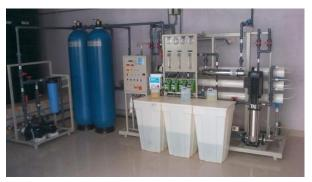
Image 2: Reverse Osmosis Water Treatment Plant installed by Safe Water Network India
