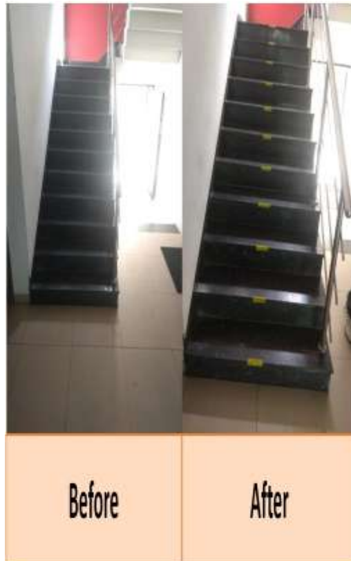
FIG 33: Photograph before and after (Steps identification)
