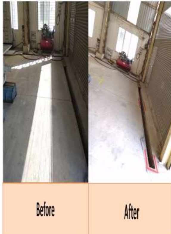
FIG 25: Photograph before and after(Marking for danger area)
