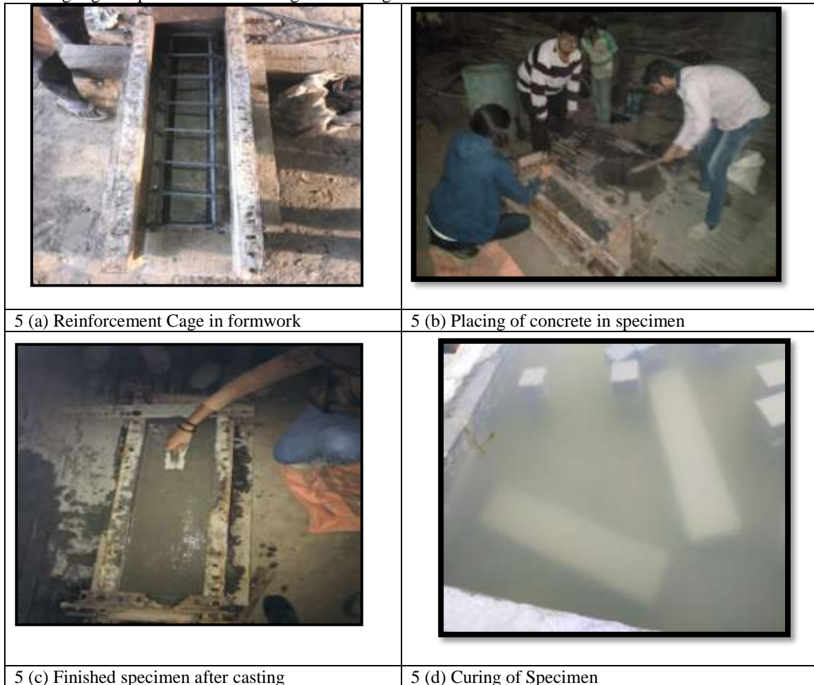
Fig. 5 Different stages of casting RCC and BFRP beam
