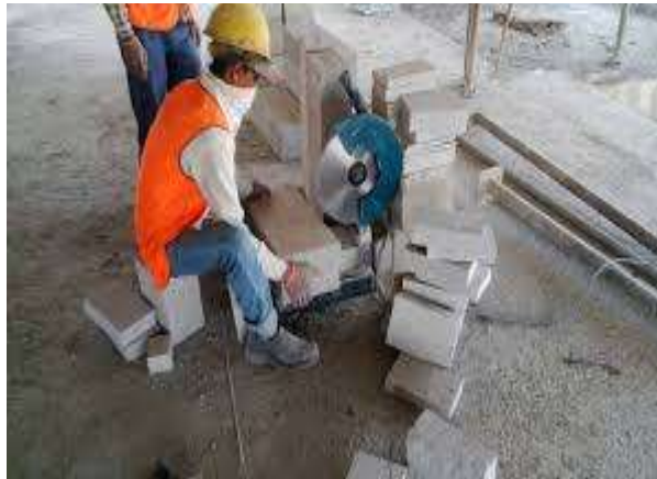
Fig: Cutting of AAC block
