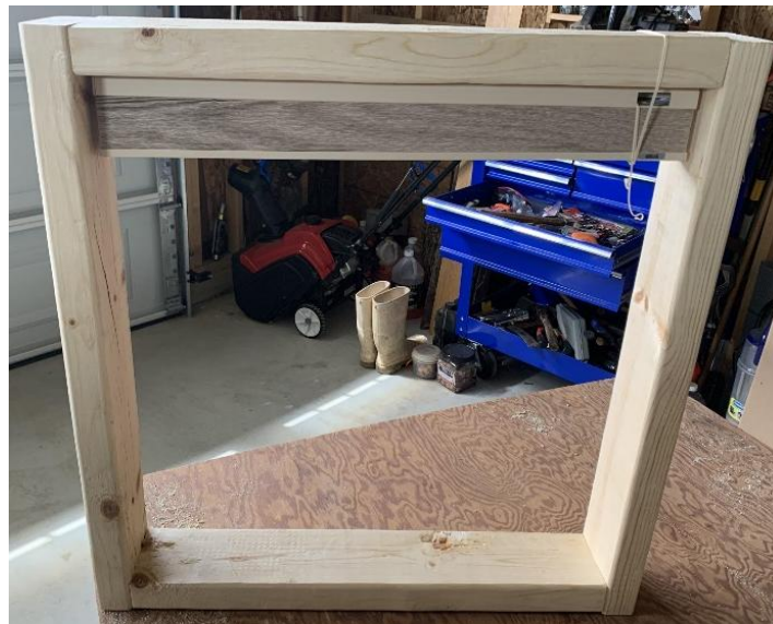
Figure 2: The frame for the blinds with blinds installed and brought up to the top.
