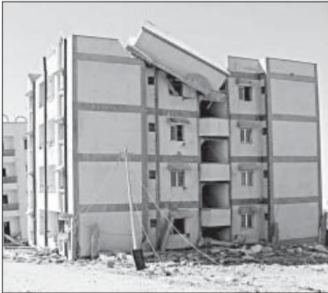
Fig 1. Failure of overhead tank in Bhuj earthquake, 2001
