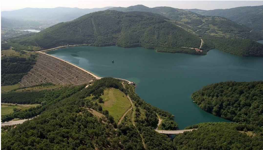
Fig. 2 –Ujmani's Dam,a rock-filled embankment dam on the Ibar River in the District of Mitrovica,Kosovo[6]
