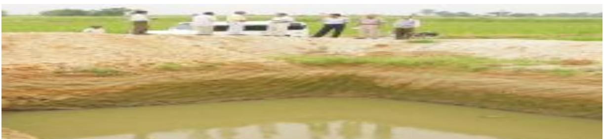
Fig.3.Excavation of farm pond
