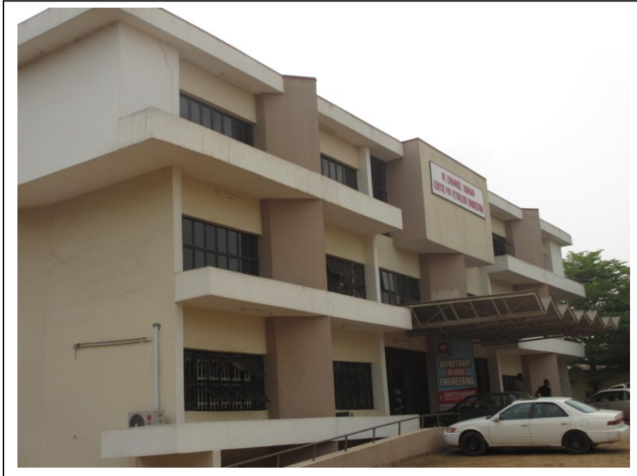
Plate 1: Photographic front elevation of Building under study
