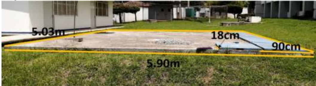
Figure 1. Cistern for rainwater collection of building A, of the ITSSNP
