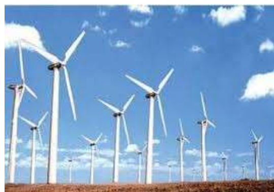
Fig. 3. A wind farm of horizontal wind turbine
