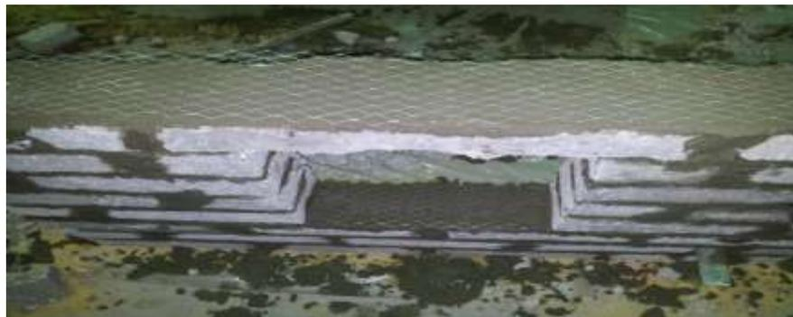
**Figure 7.** Strengthening brick walls with opening using three horizontal plies of steel wire mesh embedded into bed joint mortar (two plies above lintel and one ply at sill level)
