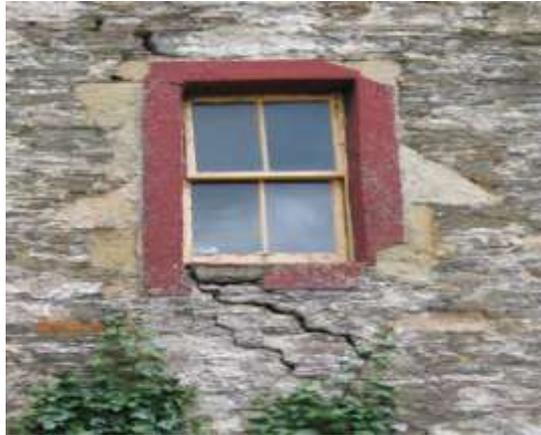
**Figure 1.** Cracks around window opening By Ingal Maxwell Published by Technical Conservation Group
