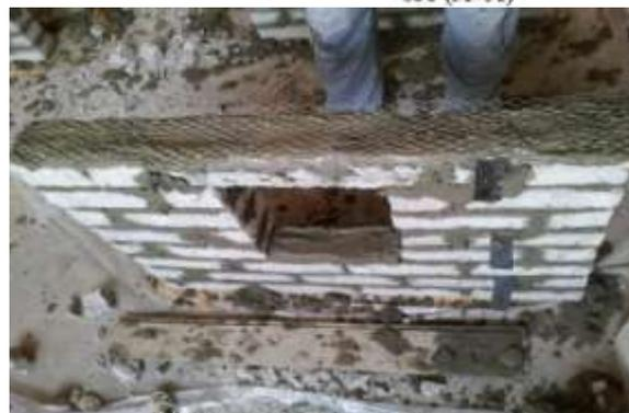
**Figure 5.** Strengthening brick walls with opening using one horizontal ply of steel wire mesh embedded into bed joint mortar above lintel.
