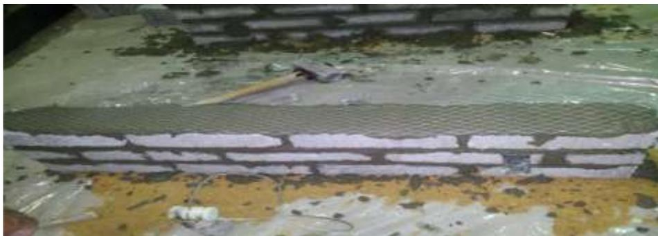
**Figure 8a.** Strengthening brick walls with opening using four horizontal plies of steel wire mesh embedded into bed joint mortar (two plies above lintel and two plies at sill level )
