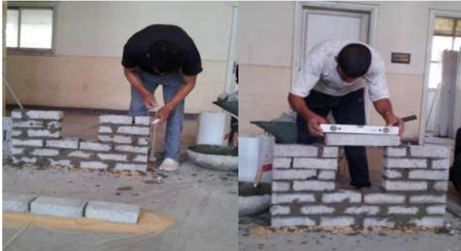
**Figure 3.** Brick wall specimen during construction
