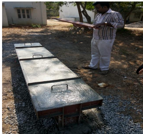
Fig 4: Concreting of Tee beam mould
