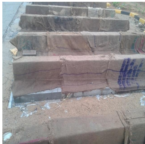
Fig 6: RC Tee Beams under Curing
