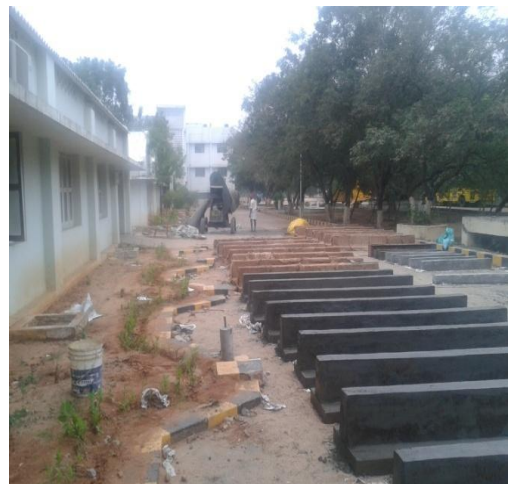
Fig 5: Demoulded RC Tee Beams
