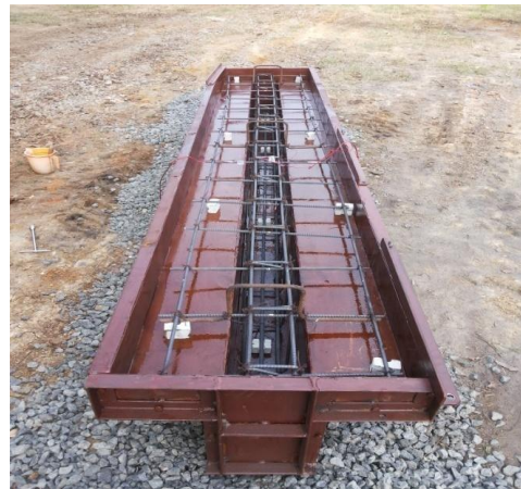
Fig 2: Tee beam mould before casting
