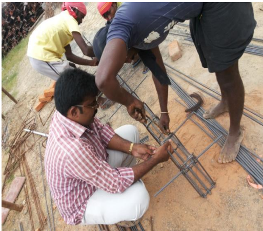
Fig 1: Preparation of Steel Reinforcement for Beams.
