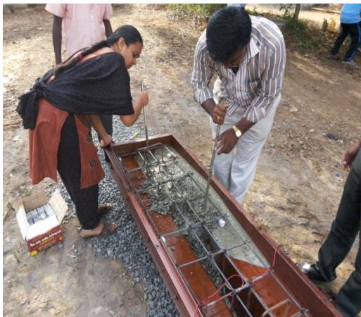
Fig 3: Pouring of Concrete on Tee Beam Mould
