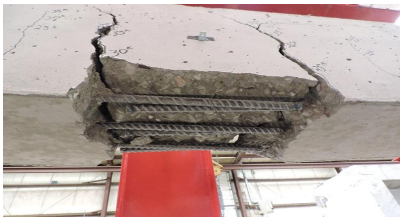
Figure 5: Typical bond failure in beam splice specimen
