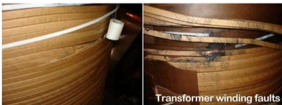
Fig 7 winding at faulty condition
